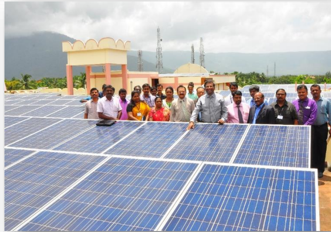
95 kW Grid Tied Solar Power Plant in Administrative Block
