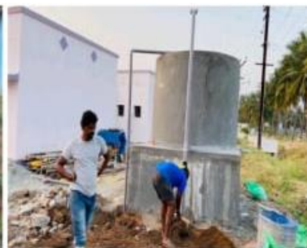
Drinking water tank construction and distribution
