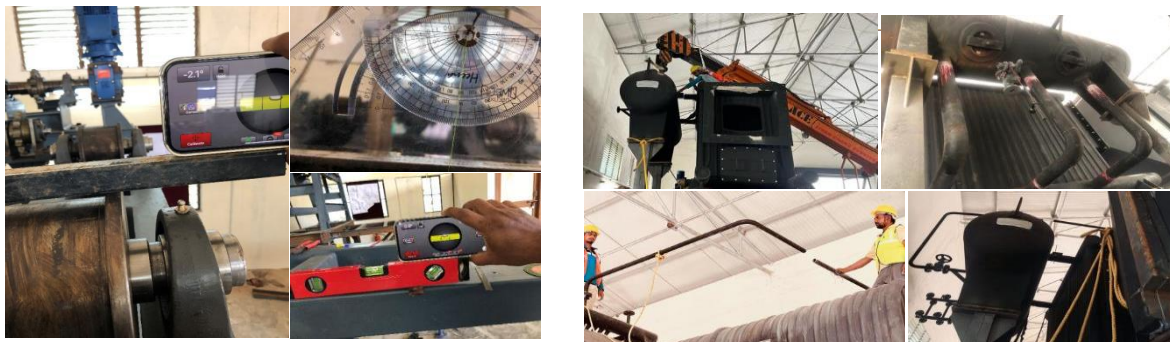
Checking of Kiln chamber alignment Steam Drum Installation and Feed Water Piping
