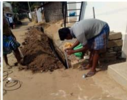
Installation of pipe line
