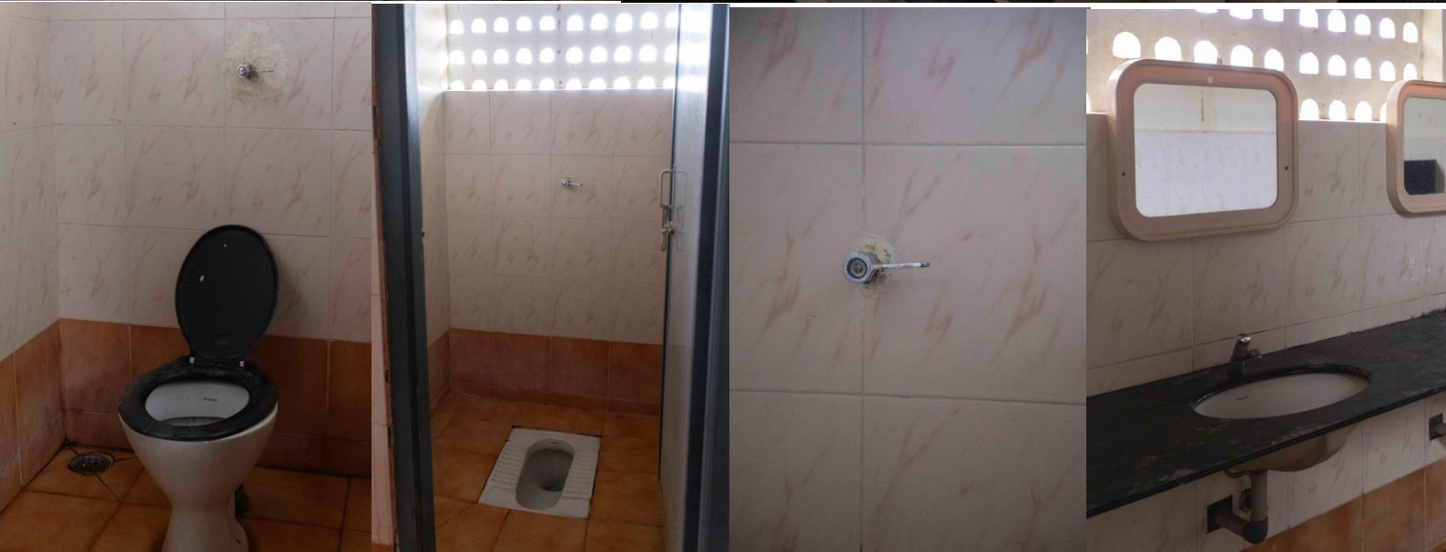
Water Efficiency Appliances (Push tap in wash basin, Hand shower, Push tap in water purifier, Flush tap) in Student Residences /Hostel and Campus
