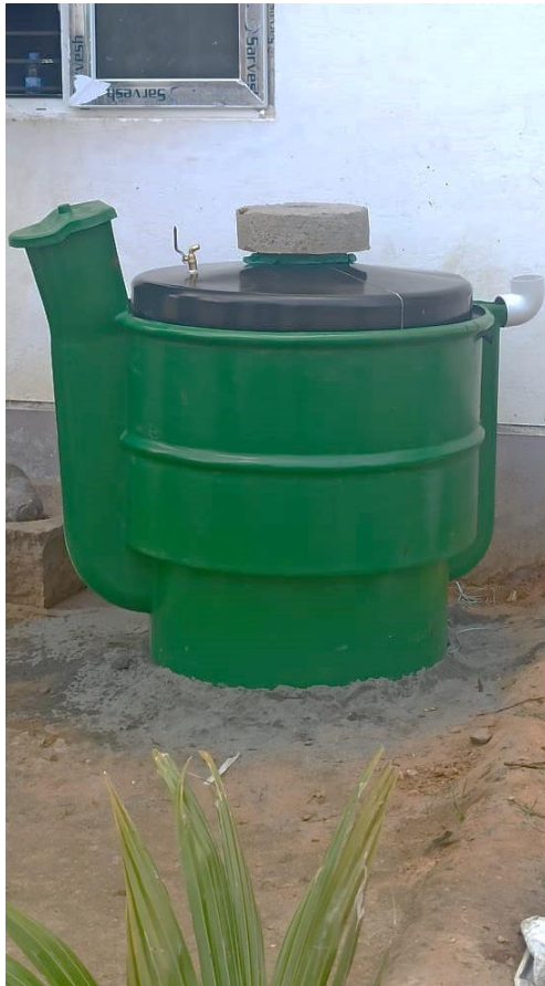
Household Biogas plant
