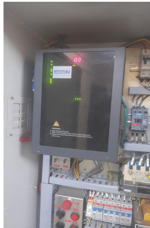
Fig 8. V3f drive based energy efficient Lifts
