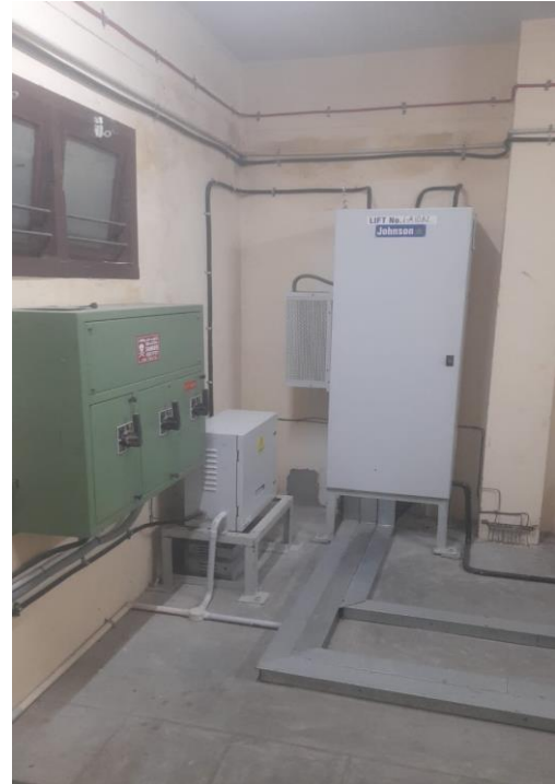
Fig 7. V3f drive based energy efficient Lifts
