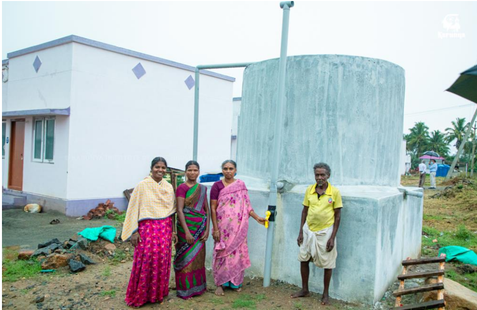
Ferrocement Tank constructed by KITS
