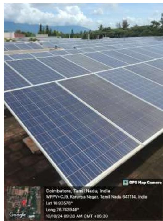
Fig 5.95kW Solar Power Plant in Admin Block: 87,473.71 kWh
