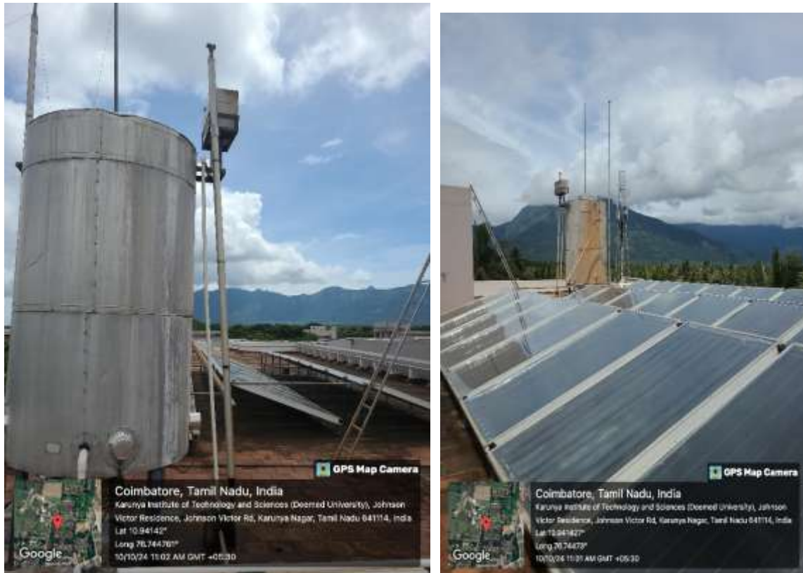
Fig 7. 87,600 LPD Solar Water heating system (30 Nos): 15,45,718 kWh
