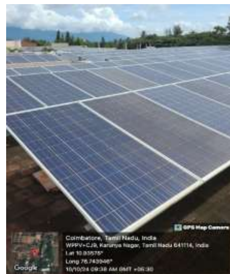
95kW Solar Power Plant in Admin Block: 87,473.71 kWh
