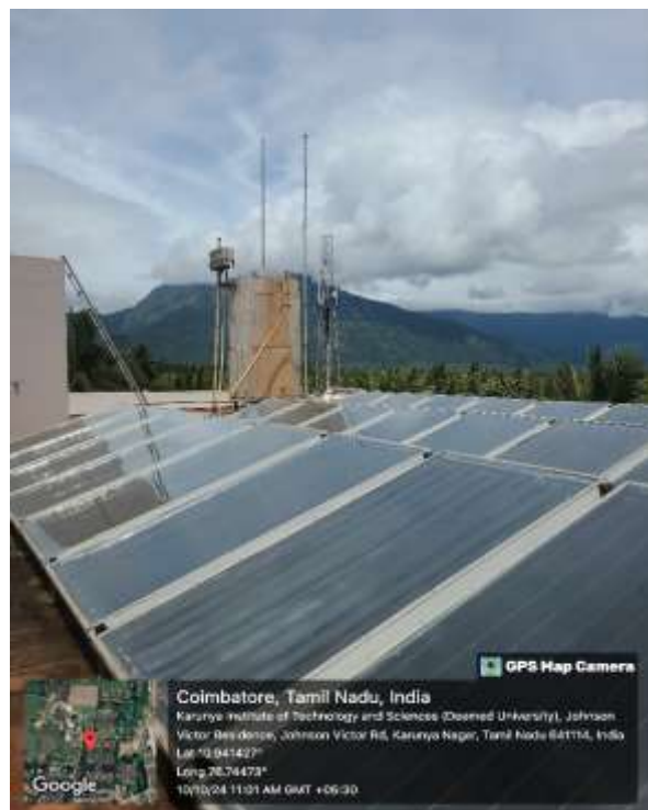
87,600 LPD Solar Water heating system (30 Nos): 15,45,718 kWh
