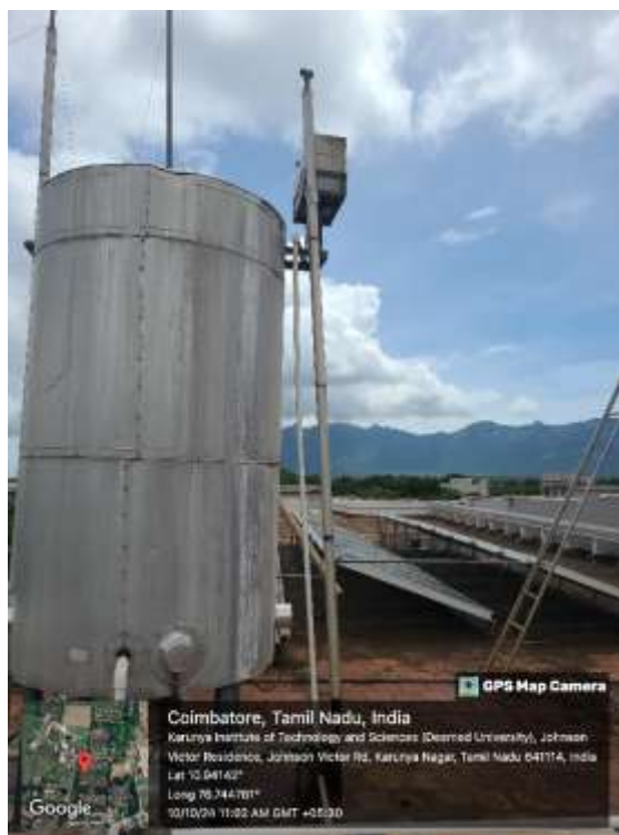
87,600 LPD Solar Water heating system (30 Nos): 15,45,718 kWh
