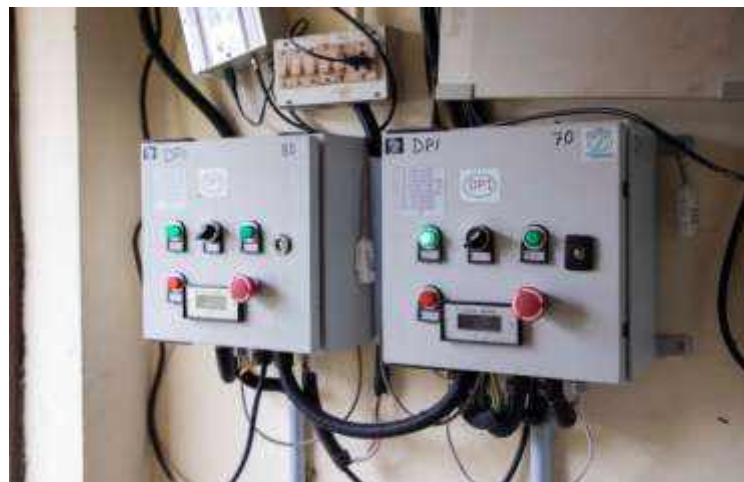
Wireless automatic water flow controllers
