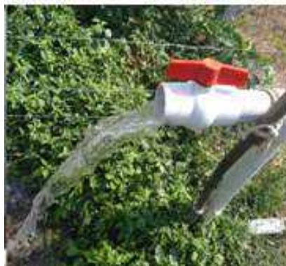
Outlet for the recycled wastewater from STP
