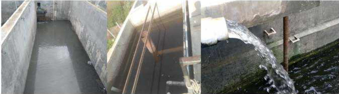
JMR Collection Tank, Settling Tank (after filtration)
