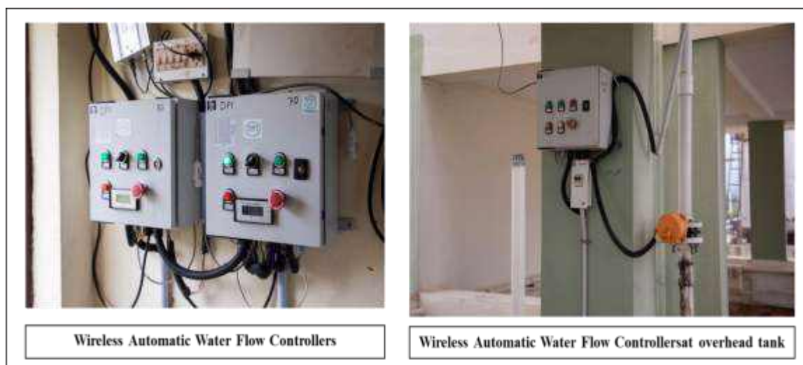
Sample pictures of Wireless automatic flow controllers in the campus
