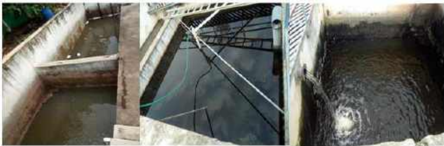
FDR Collection Tank, Settling Tank (after filtration)
