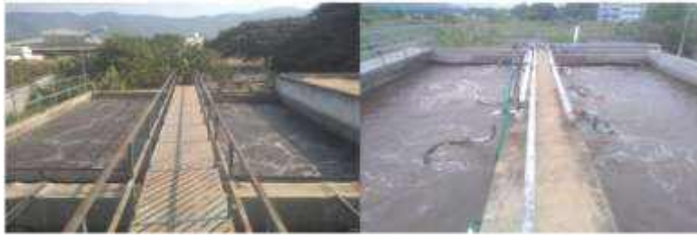
JMR and LH STP – Aeration Tanks
