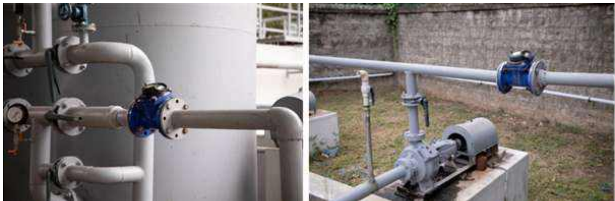
Flow Meters at the Filter Unit of Treatment Plant to measure the Treated Water
