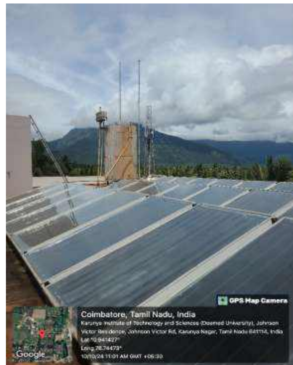
87,600 LPD Solar Water heating system (30 Nos): 15,45,718 kWh
