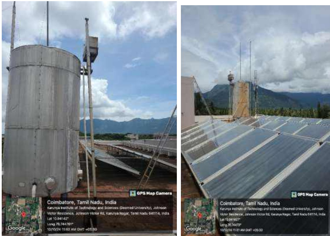
Fig 7. 87,600 LPD Solar Water heating system (30 Nos): 15,45,718 kWh
