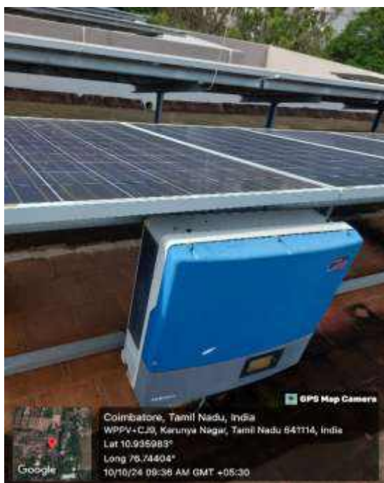
Fig 5.95kW Solar Power Plant in Admin Block: 87,473.71 kWh
