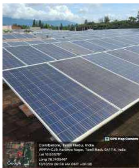
95kW Solar Power Plant in Admin Block: 87,473.71 kWh
