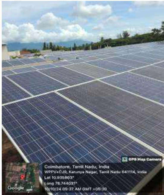
20kW Solar Power Plant in EVR/Oprah Mess Building: 24,388 kWh
