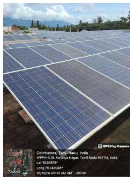
Fig 5.95kW Solar Power Plant in Admin Block: 87,473.71 kWh
