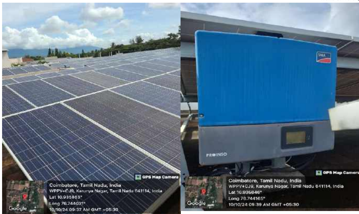
20kW Solar Power Plant in EVR/Oprah Mess Building: 24,388 kWh
