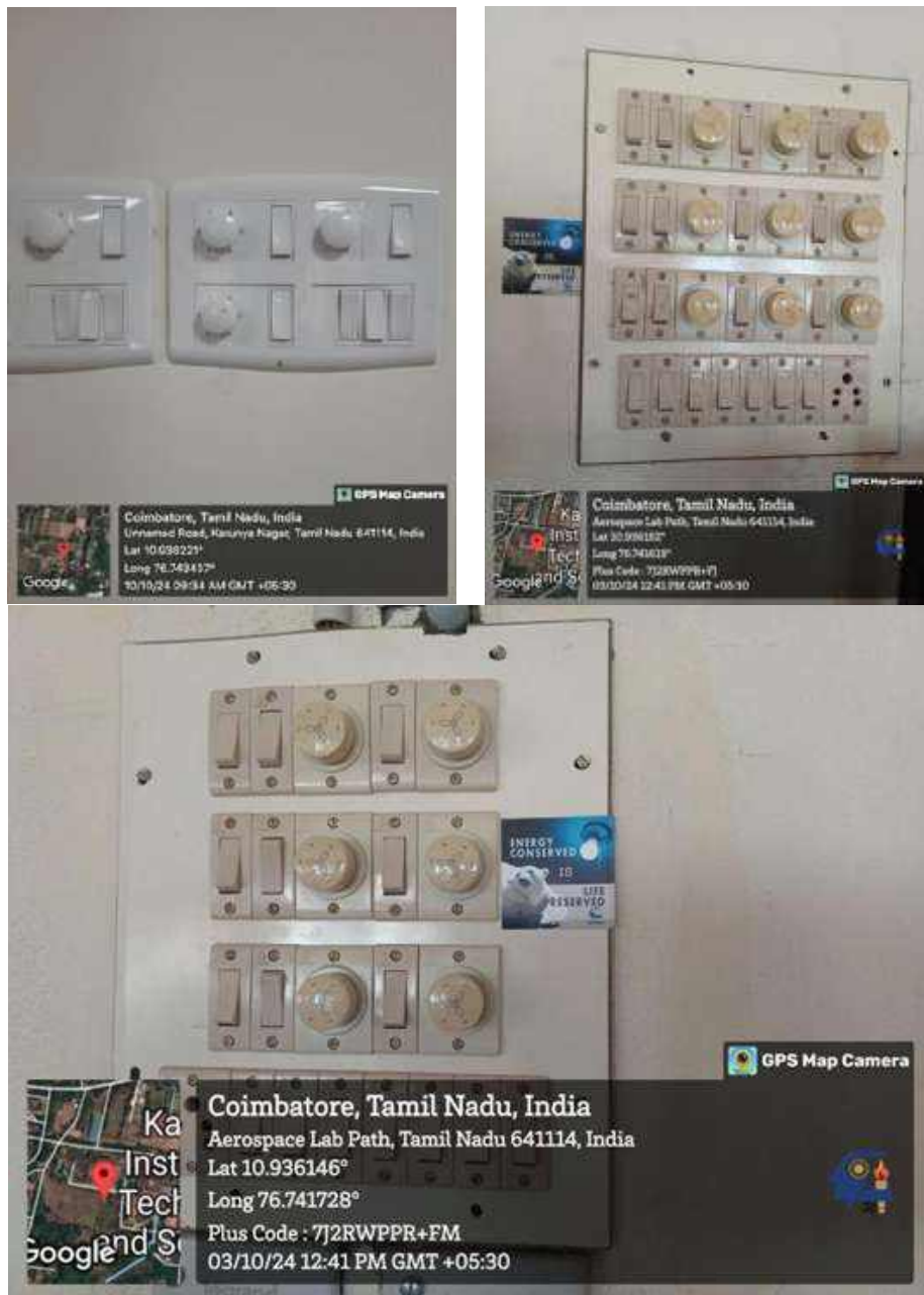
Electronic Fan Regulators in place of Electric fan regulator for Power savings across the campus
