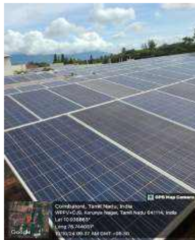
95kW Solar Power Plant in Admin Block
