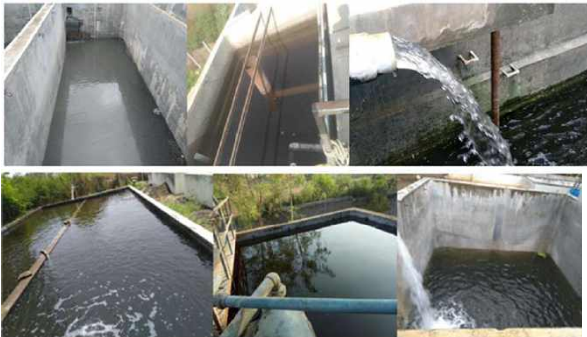
Storage tanks for treated water (before reuse in the garden)
