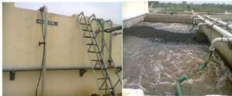
Fluidized Bed Bio-Reactor
