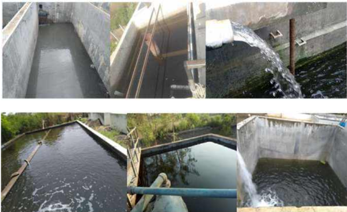
Storage tanks for treated water (before reuse in the garden)
